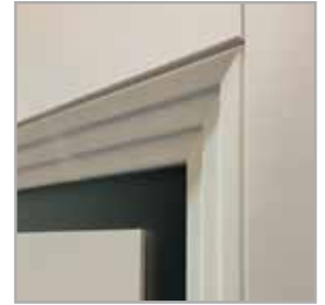
panel with finished edge glued to the glass – version V1SP
