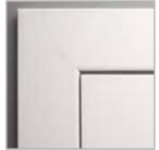
architraves connected in a standard way at an angle of 45° for the DIN DUO door frame
