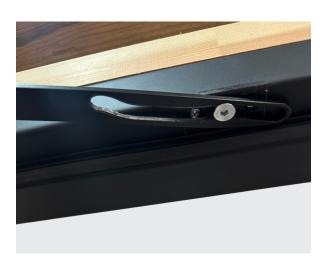
Designed for interior entrance doors, including fire doors, on wooden or metal frames. It is a more economical alternative to a concealed door closer. Adjustment is made by tensioning the spring, which regulates the closing force.
