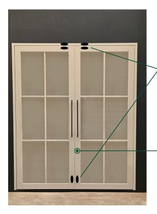
Closed with magnetic catches located in the door leaf and frame
