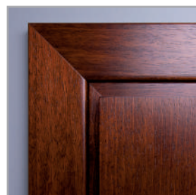
interconnection of architraves at an angle of 45°
